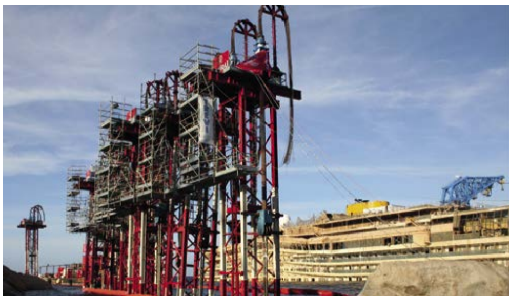
Costa Concordia recovering project. (ph. credit Trevi)
