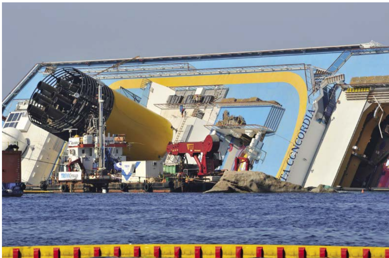
Costa Concordia recovering project. (ph. credit Trevi)
